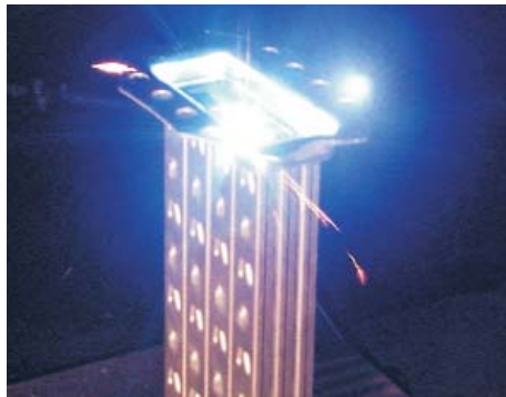
Fig. 2b: Welding of the duct-bottom-joint at the exhaust heat exchanger utilizing CO 2 laser, gantry machine, and beam deflecting optics
